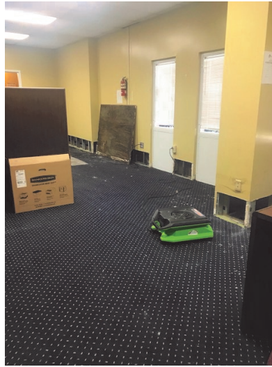
Before repairs to the walls
