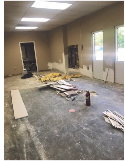
Carpet removed and walls are in the process of being painted
